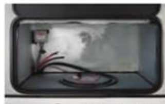
Generator Prep (Standard 27 KB, 29 SS)
